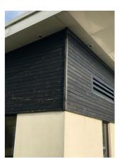
Parts of the cladding around the church building is falling down. Quotation of cost to replace wooden cladding with UPVC (plastic) £4,500
